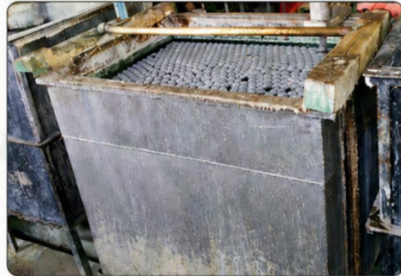
AFTER: Cathodic Cleaning tank
